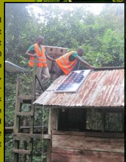
One of Tusk Trust’s new solar panels being installed
